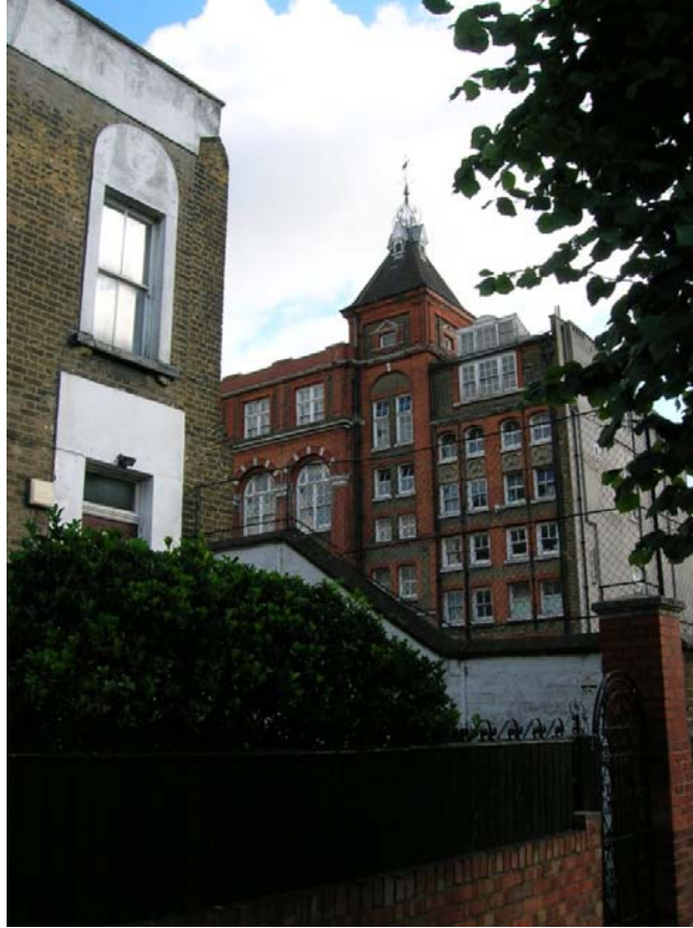
Figure 19: No. 1, Albion Drive and the former Queensbridge Board School
