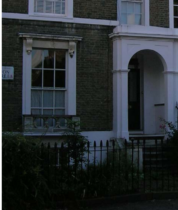
Figure 35: Replacement balconies in concrete in Albion Square
